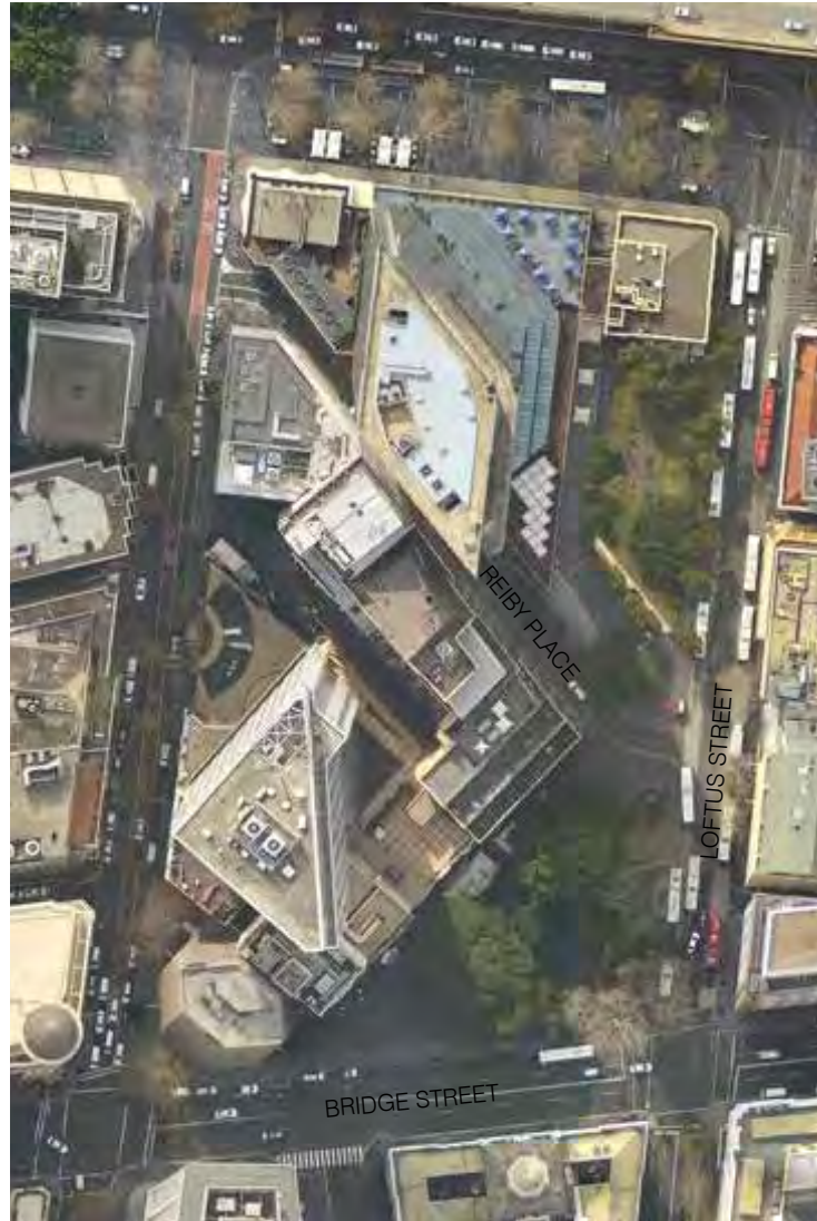
Loftus Street and Reiby Place - existing
